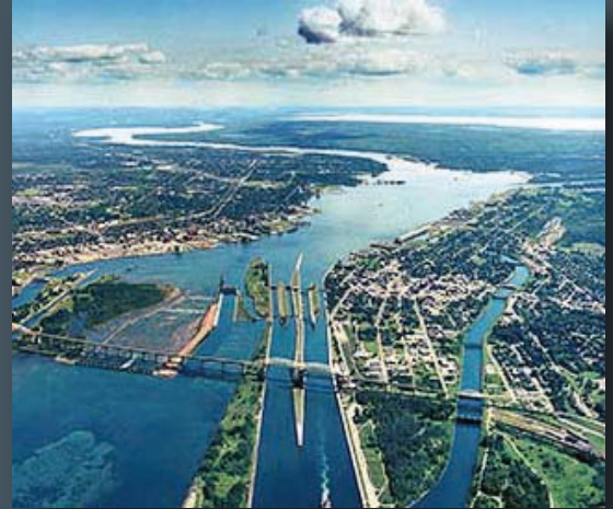
Soo Asset Recapitalization Project
